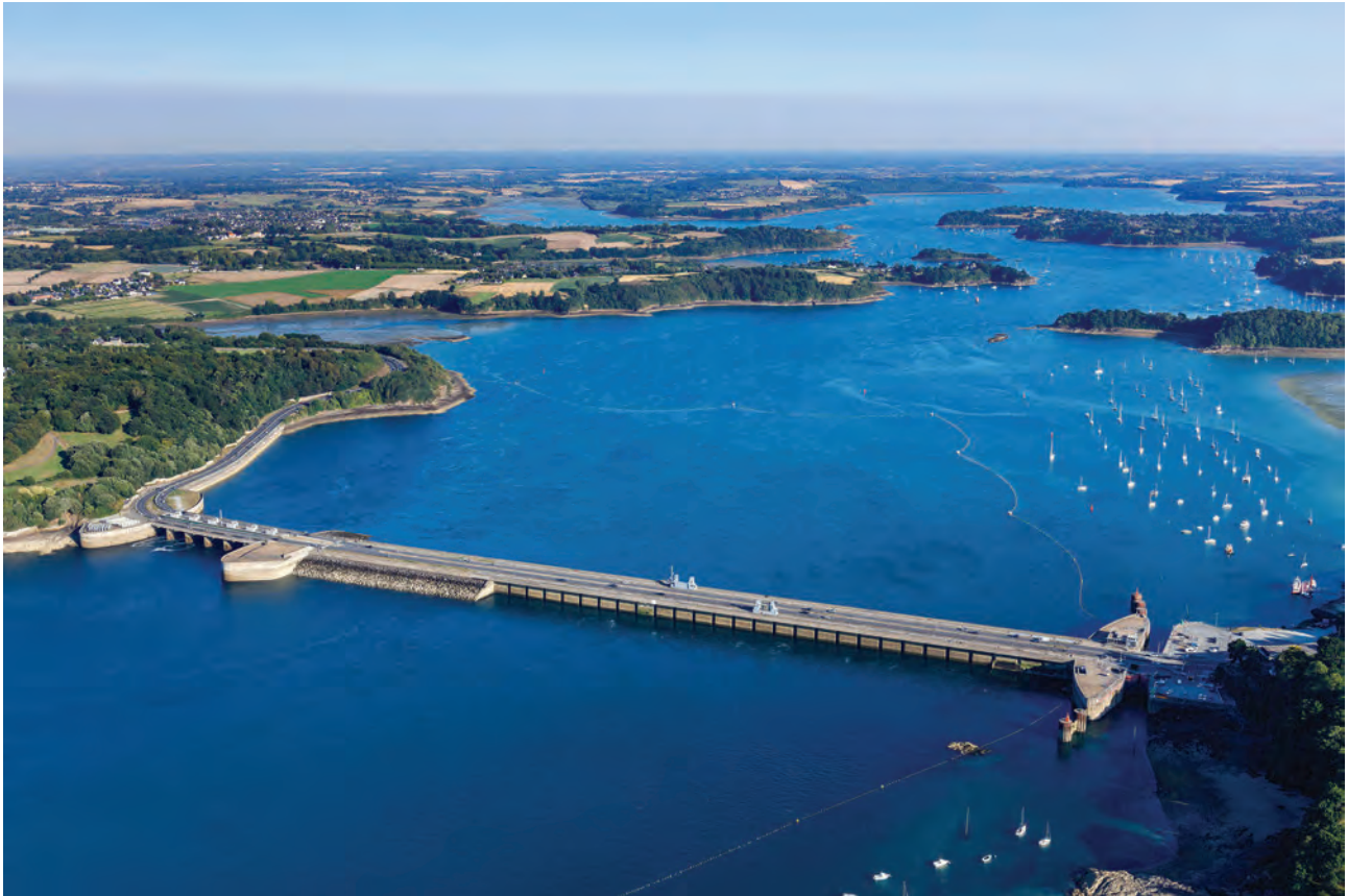
Fig. 8 – The Rance tidal power scheme, Brittany, France
