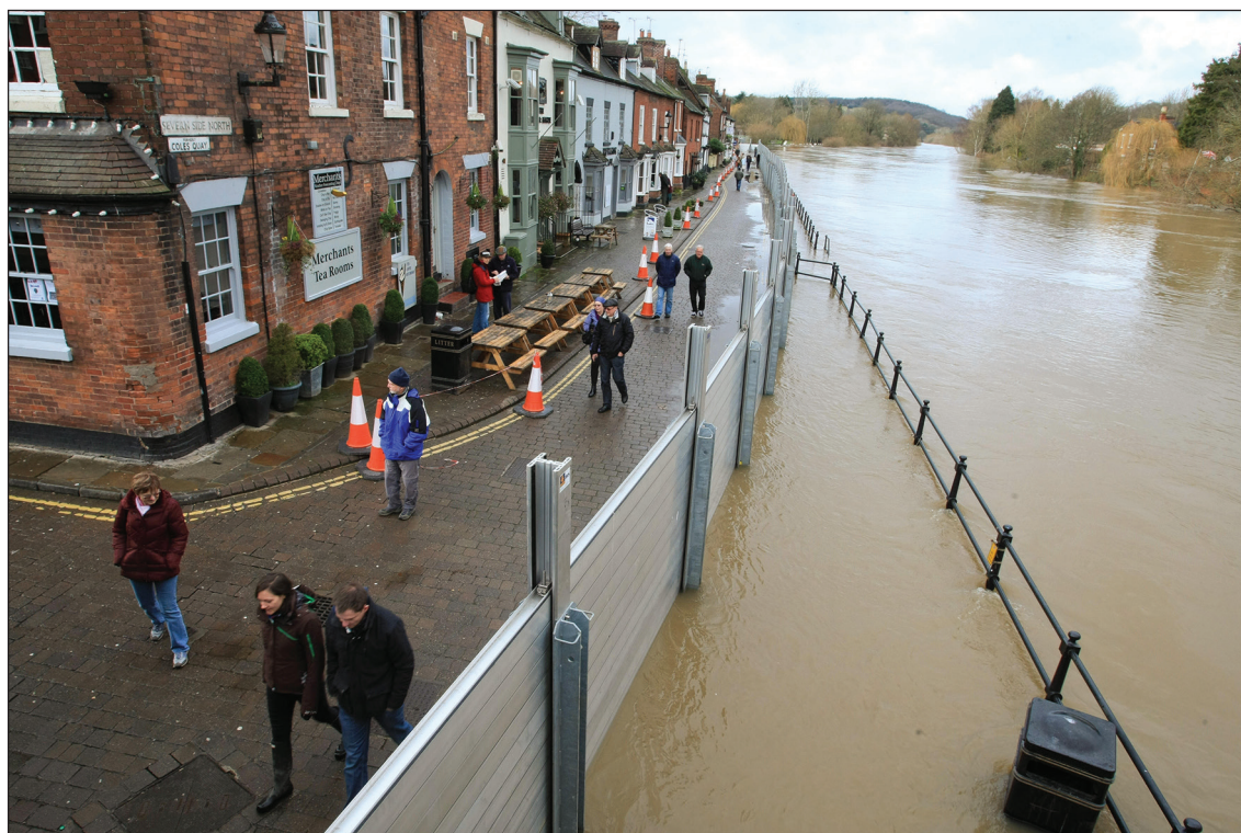
Photograph 2.1 - A flood event in Bewdley
