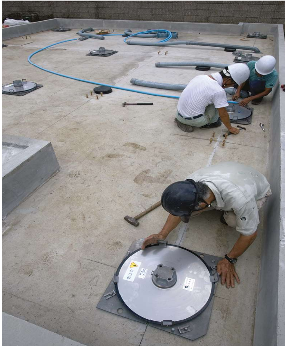
Workers install ball bearing slides to earthquake-proof a house
