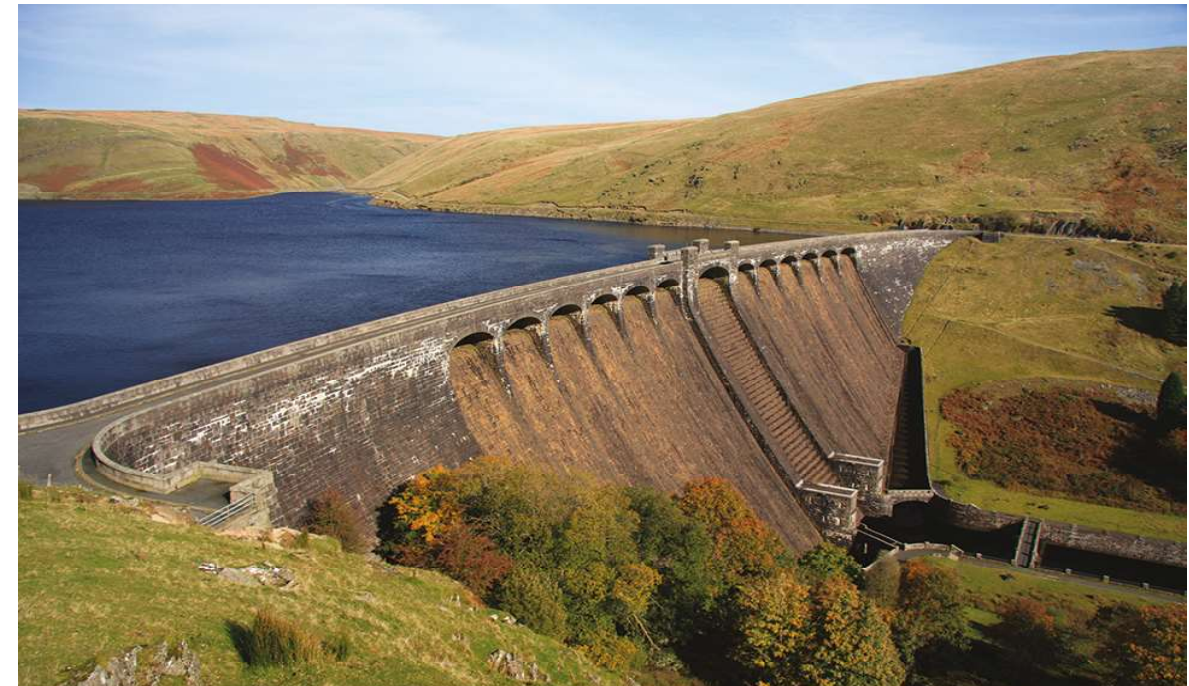
RESERVOIR AND DAM IN WALES
