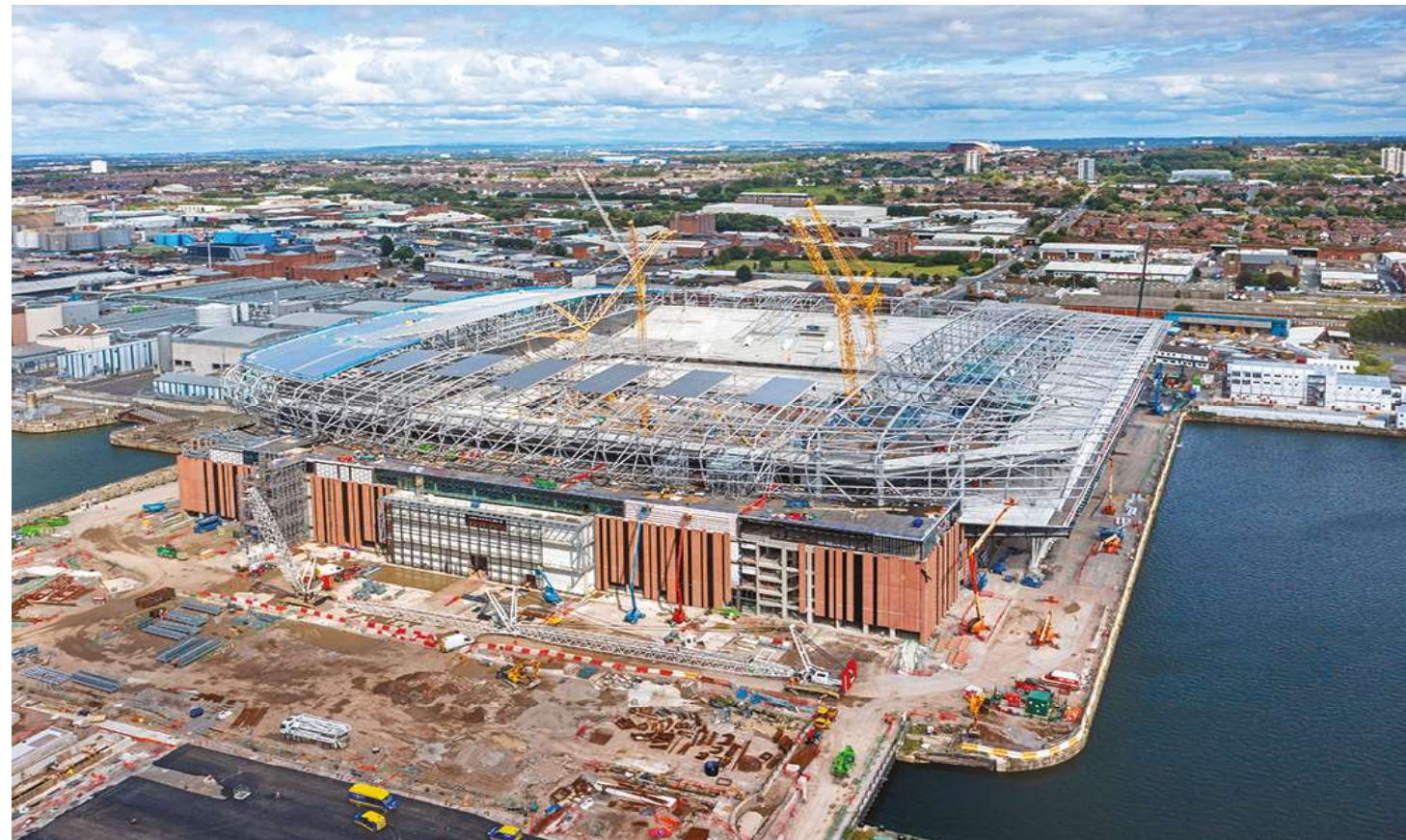
Building the new Everton Football Club Stadium
