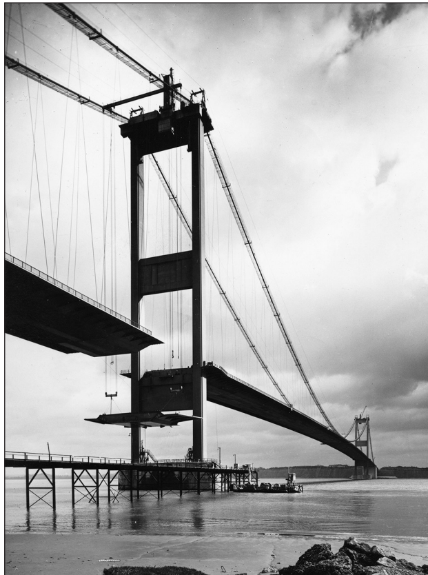
[A photograph of the final stages of building the Severn Bridge connecting the new M4 motorway between England and Wales, 1966]
