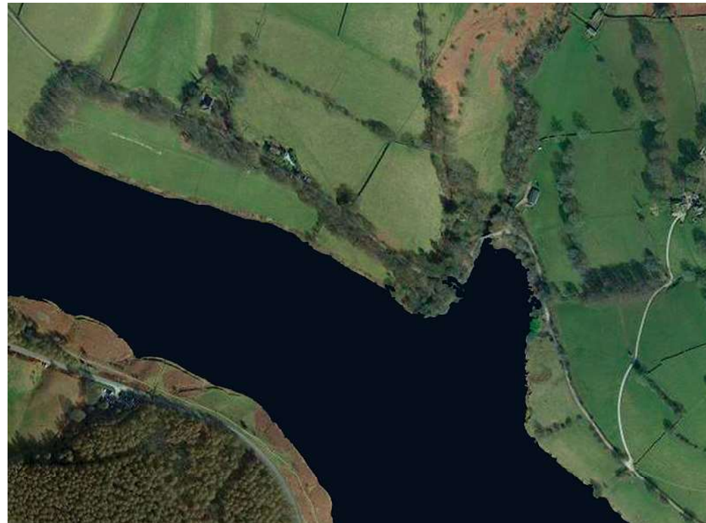
Aerial photograph of the reservoir (2024)
