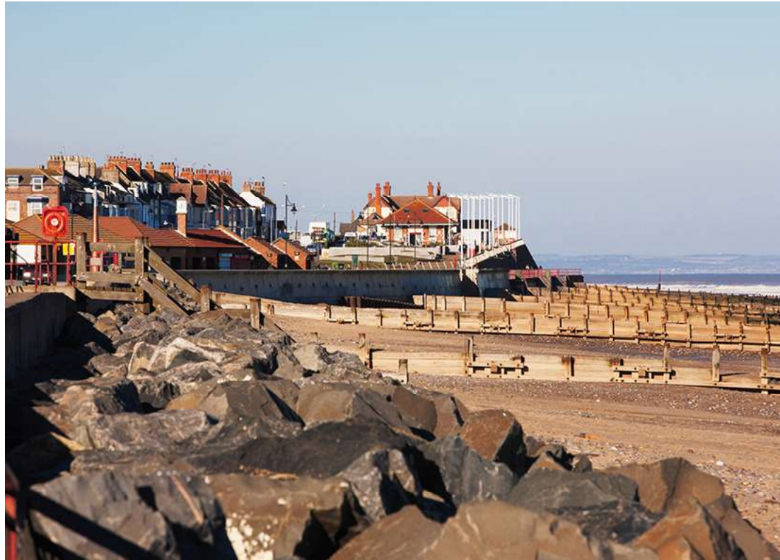
FIGURE 9a: COASTAL PROTECTION, HORNSEA, YORKSHIRE
